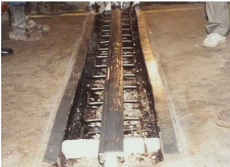
PHOTO 7 – Expansion Joint Replacement
