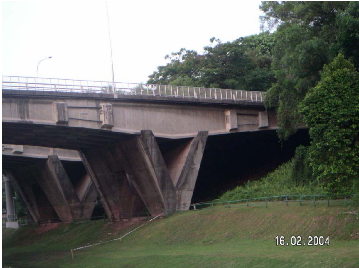
PHOTO 4 – External Post Tensioning
