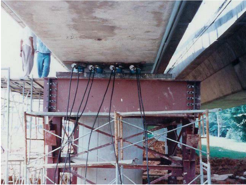
PHOTO 8- Bearing Replacement
