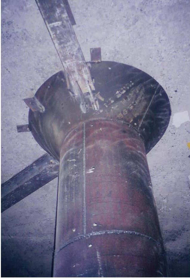
PHOTO 2 – Steel Plate Bonding
